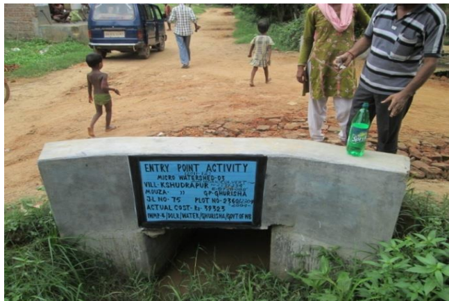
CULVERT ON DRAIN
