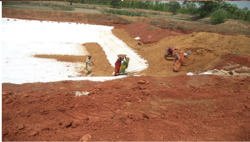
LAYING OF FIBER BASED POLYTHENE SHEET FOR PERCOLATION LOSS PREVENTION
